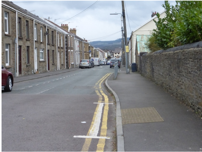
Photograph 4 – Down Street showing extended (built out) footway, pedestrian guardrail, crossing point and waiting restrictions.
